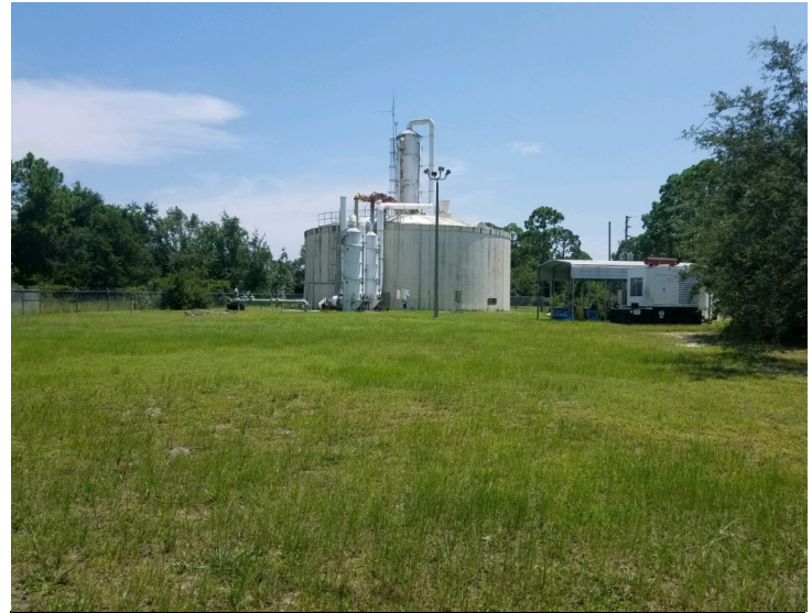
City of Apalachicola's upgraded water treatment plant.
