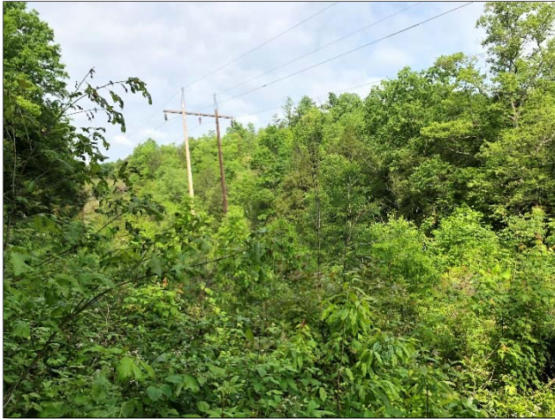
Overgrown ROW in vicinity of Laurel Creek, no herbicide
