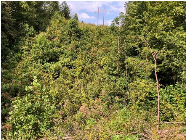
Overgrown ROW on hillside, only manual maintenance
