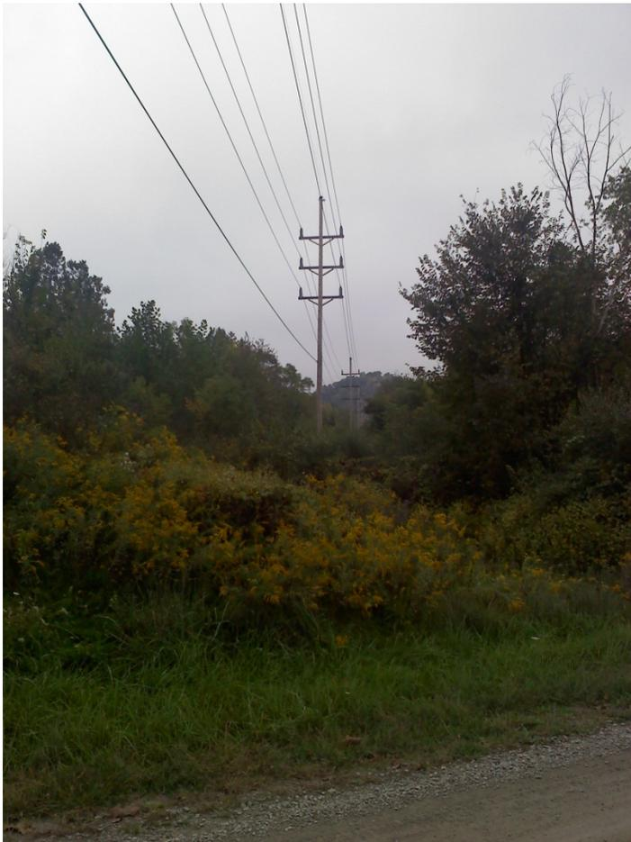
**Figure 2-16.** View south from Chapel Drive of existing 69 kV wood monopole transmission line. Proposed transmission line will immediately parallel this line to the east (left).
