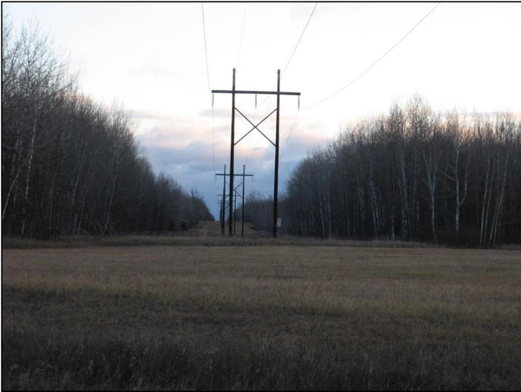
View of existing 115 kV H-frame structure along Route 1A
