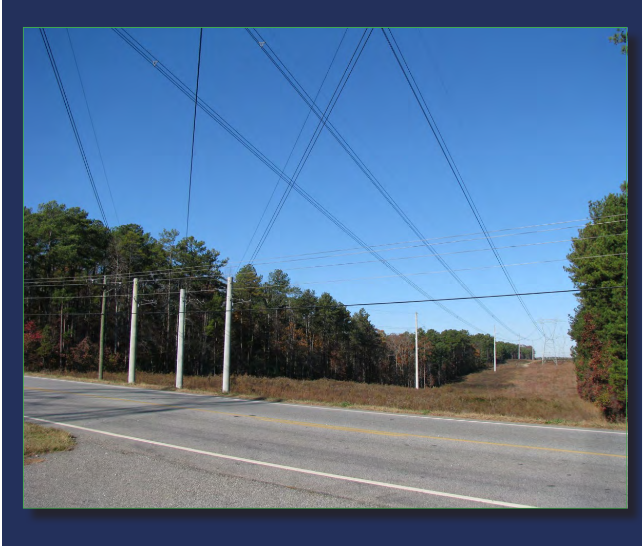
Figure 2. View of Existing 230 kV and 500 kV Transmission Lines
