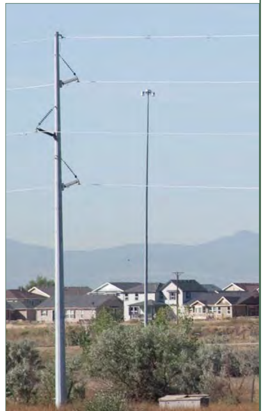
Below: Swan flight diverters on the Phase II transmission line
