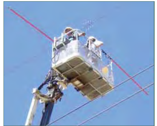
Above: Installation of swan flight diverters
