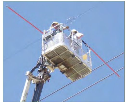
Above: Installation of swan flight diverters
