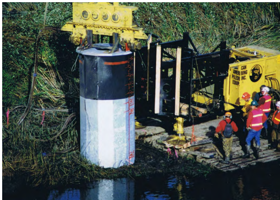
Helicopter Based Vibratory Caisson and Hammer Unit
