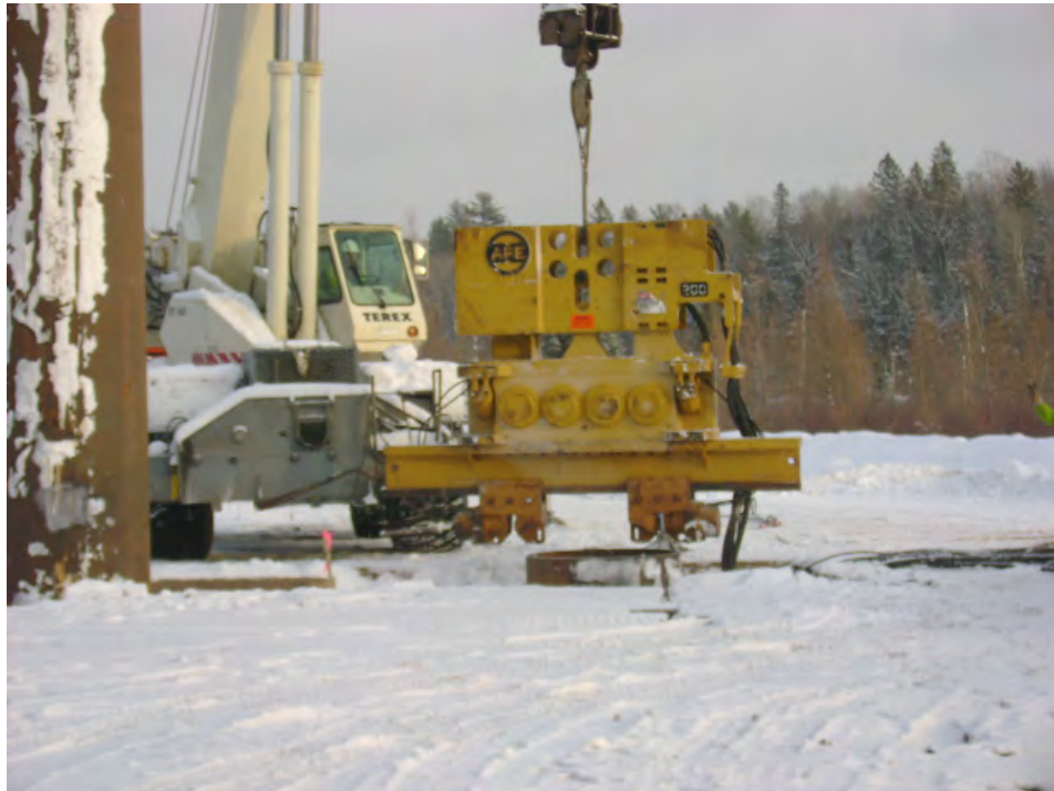
Ground Based Vibratory Caisson and Hammer Unit
