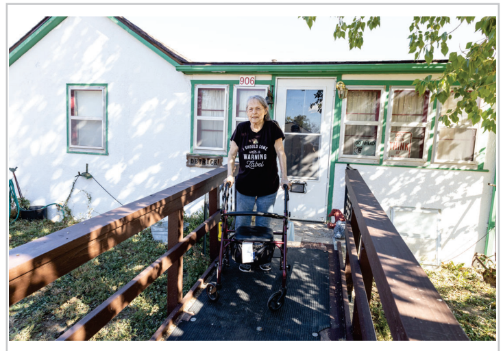
Loretta stands on her new exterior ramp funded by a 504 repair grant. She is now able to safely enter and exit her home unassisted.
