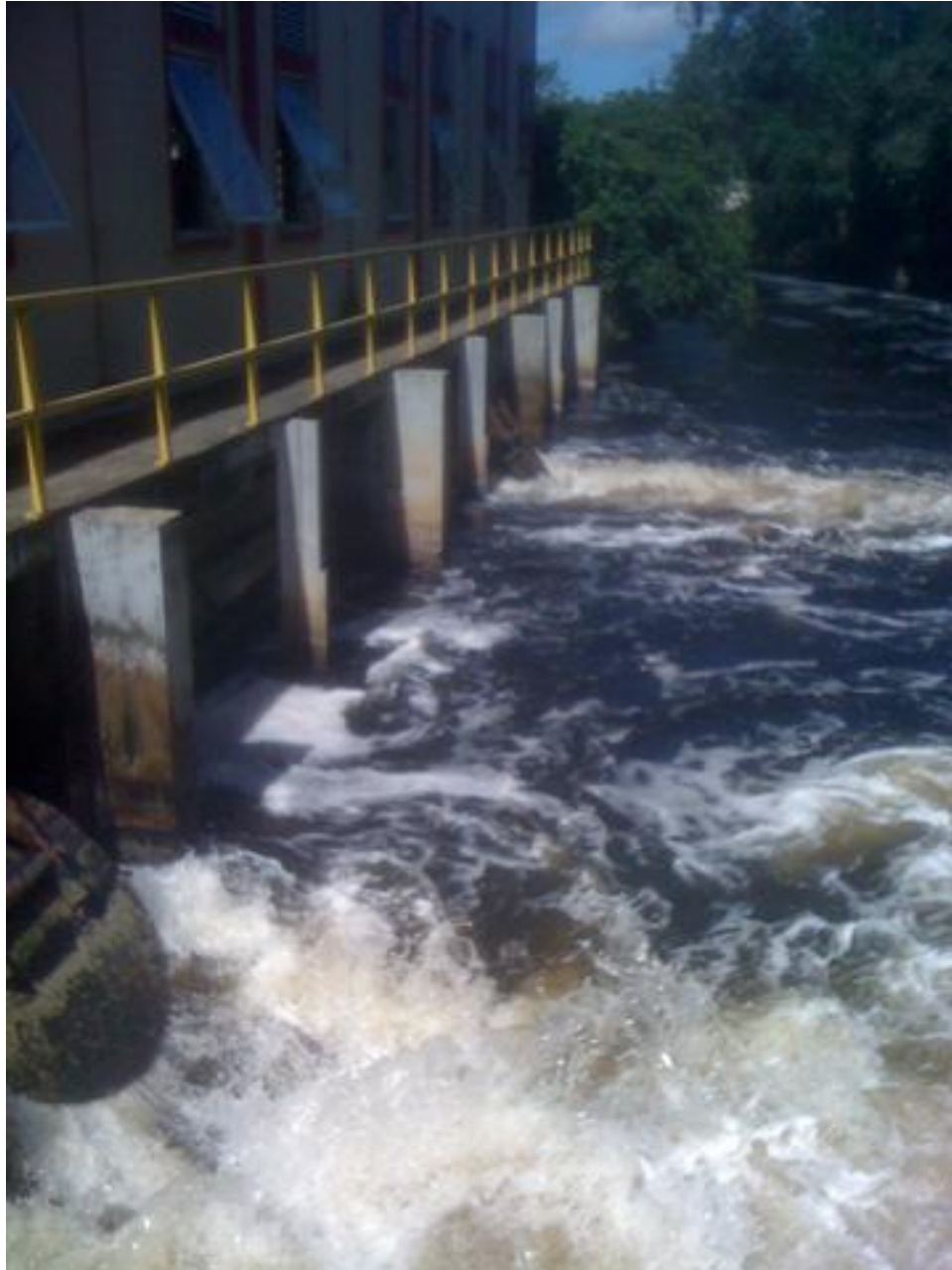
Figure 1-22: Photo of Excedent Brackish Water Discharge – El Vigía Pumping Station
