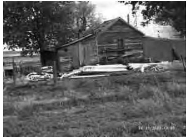
Photo #10 View of dilapidated storage shed on southern adjoining property.
