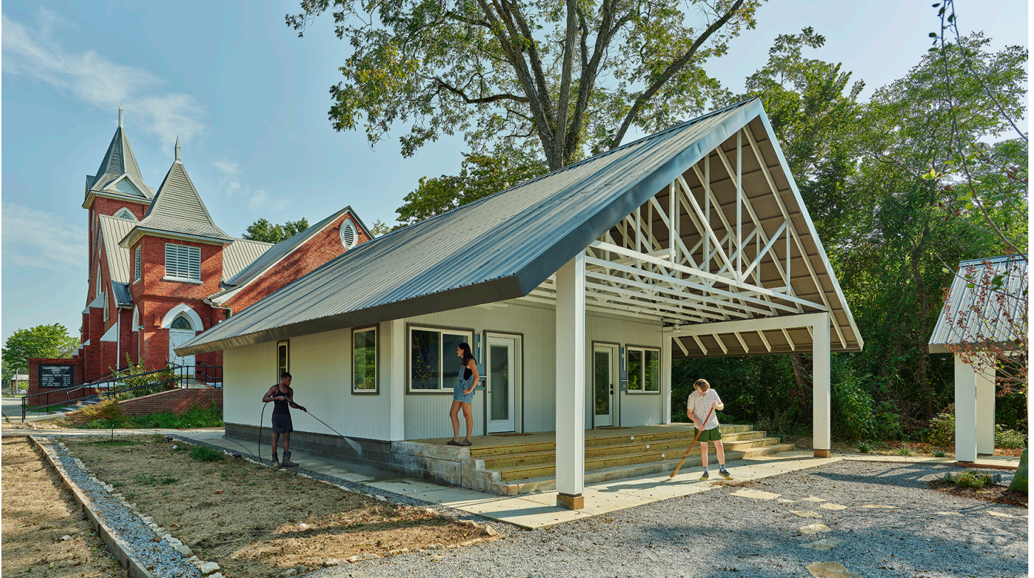
C.H.O.I.C.E. House under construction
