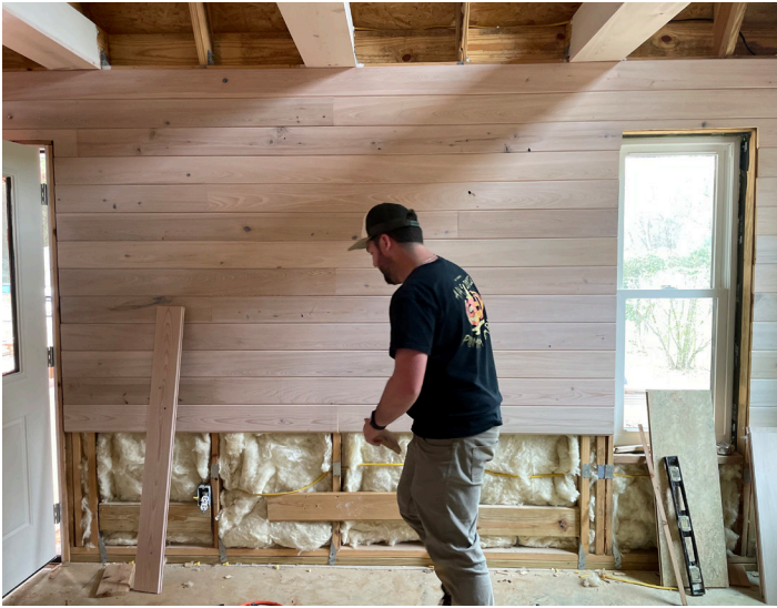
Some interior walls feature wood cladding on the wall and ceiling
