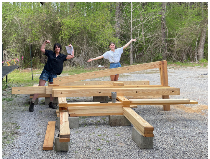
Construction mock-up on the site
