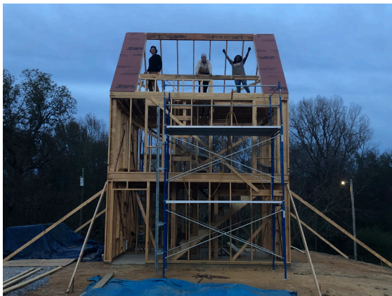
Framing the house
