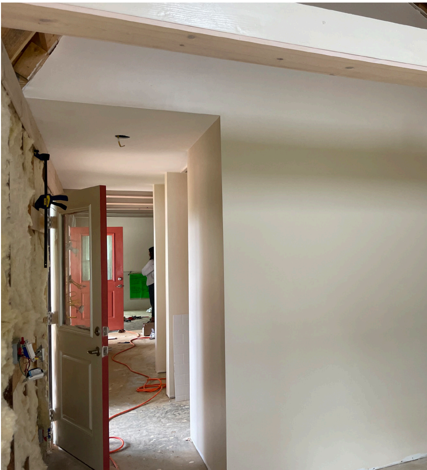
Interior finishes are being installed in the home
