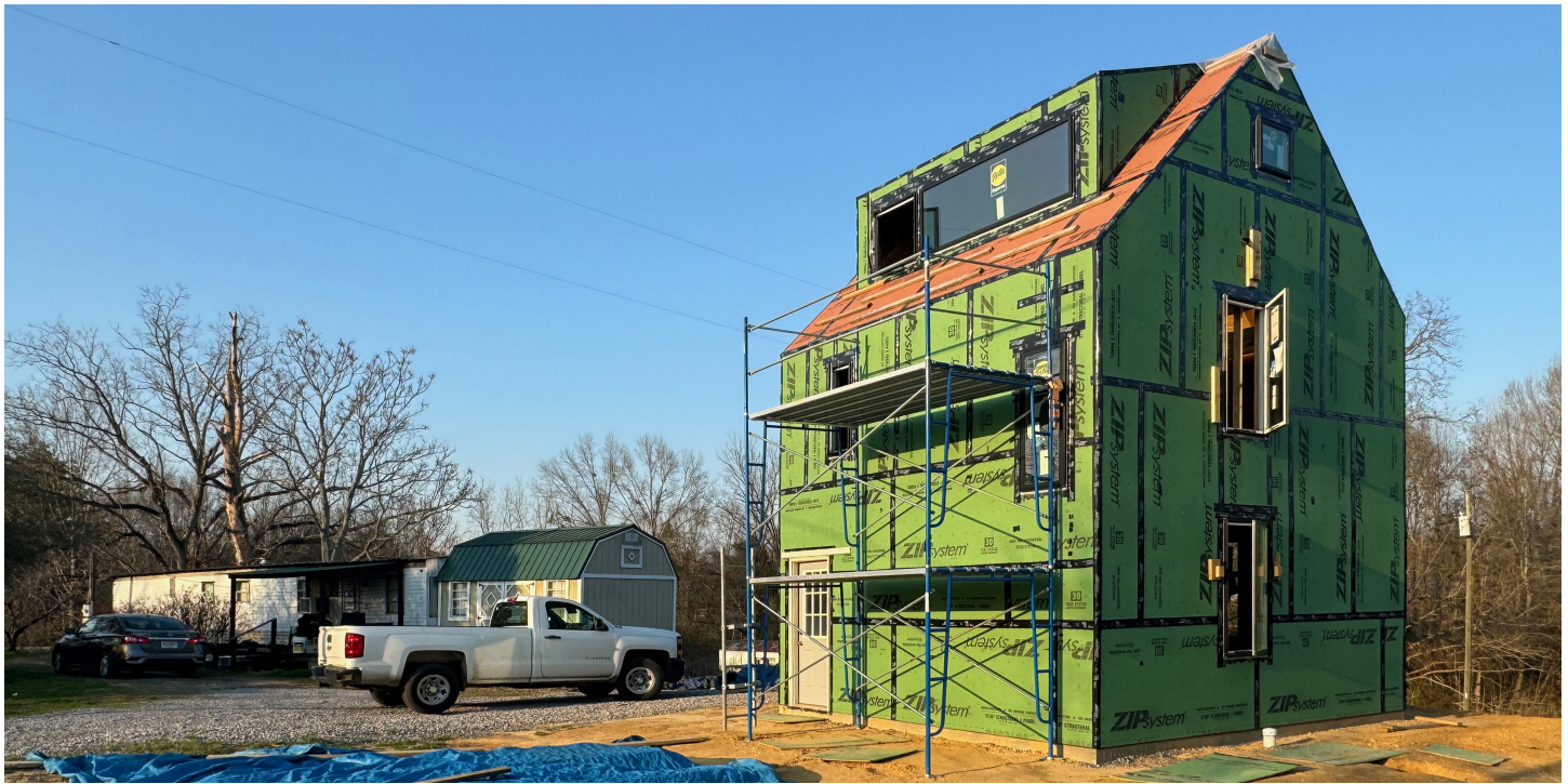
18x18 house under construction
