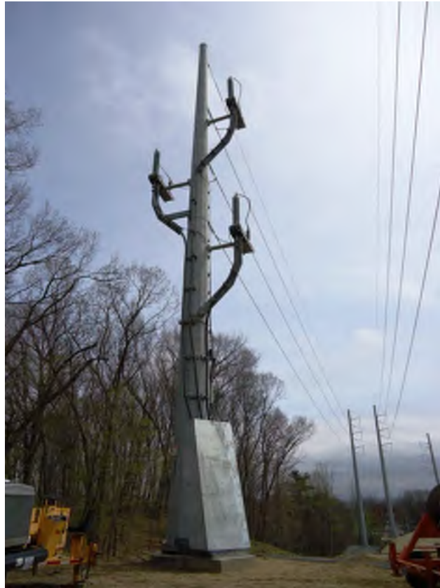
Figure 4-6: Typical 161kV Transition Structure
