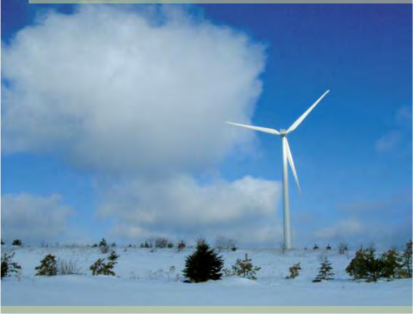
The 35 wind turbines of the Stony Creek Wind project can produce a combined 52.5 megawatts of power. Southern Maryland Electric Cooperative and Old Dominion Electric Cooperative in Virginia are purchasing power from the project. Photos courtesy Stony Creek Wind
