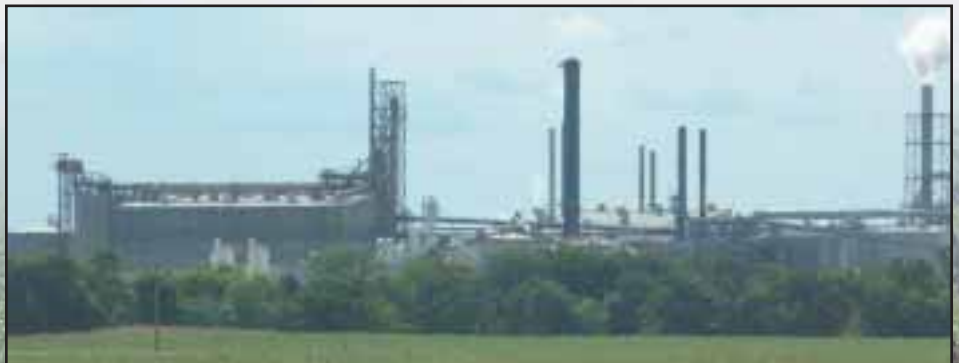
The former Minnesota Corn Processors plant, now owned by ADM, near Marshall, Minn.
