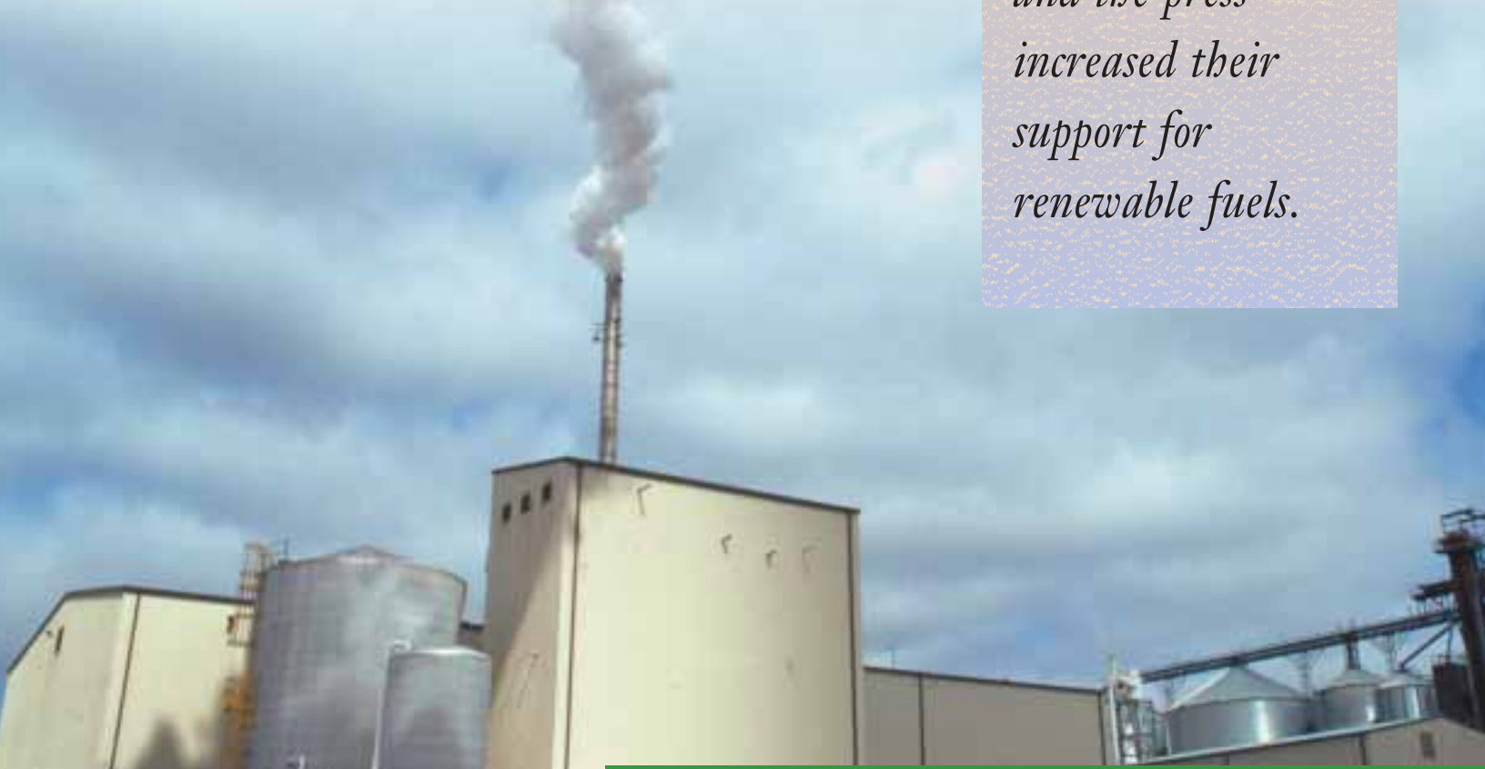
Ethanol refineries, such as this plant, should be located in an area where most of their grain needs can be secured within a 30-mile radius.
