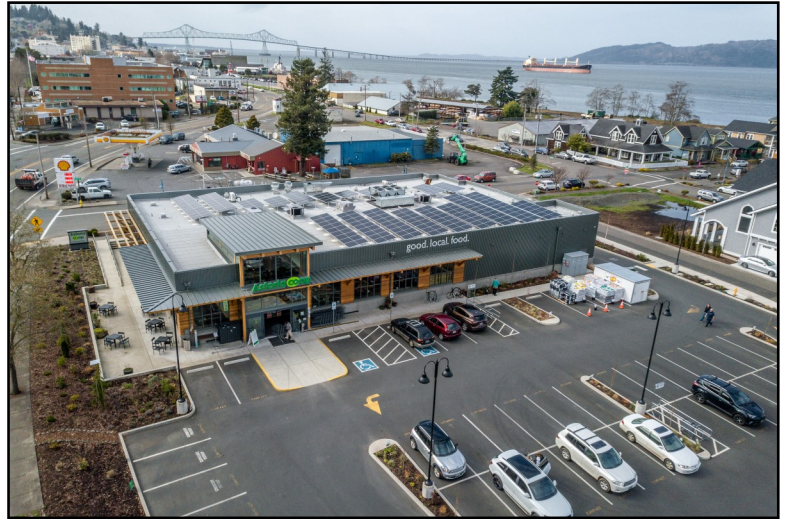
Photo courtesy of Trav Williams, Broken Banjo Photography. The Astoria Co-op installed rooftop solar panels to offset its energy use.
