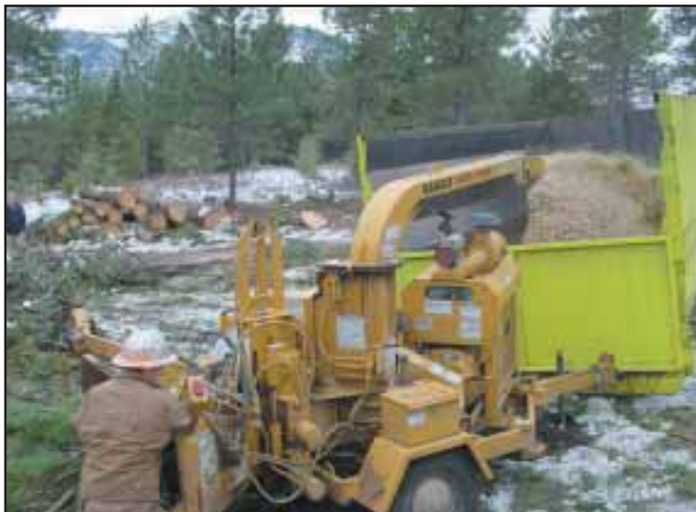
Forest thinning operations — conducted here by Horizon Tree Service and All Woody Resources — will lessen the threat of a devastating forest fire. The wood chips will provide fuel for generating electricity. Photo courtesy Montana Community Development Corp.
