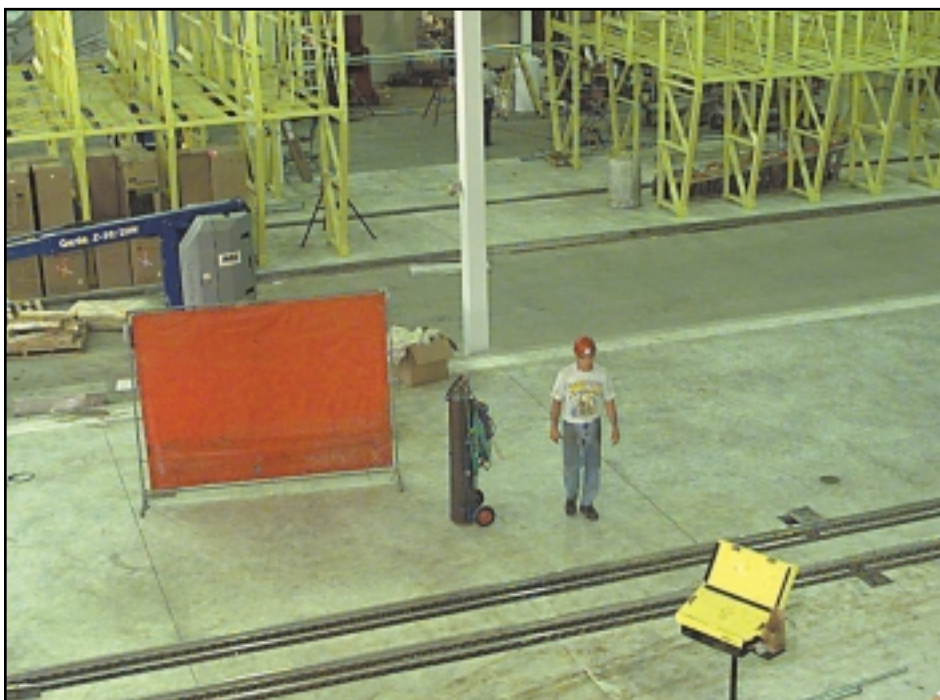
"The accident taught us that you periodically need to practice your emergency response plan, because these unpredictable things can happen," said Wally Weil, operations manager. Here, repair work proceeds to restore the co-op's milk processing operations. Photo by Patrick Ferron, courtesy Green Bay Press-Gazette
